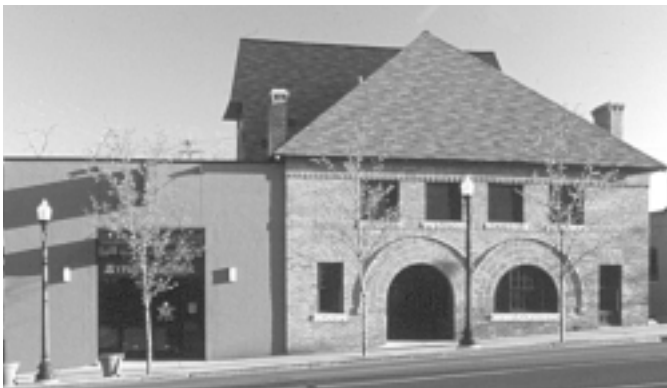
11 W. Michigan Avenue (Flour Mill ) c. 1845 Owner: Phoenix 11 121 Pearl Street #607, Ypsilanti
