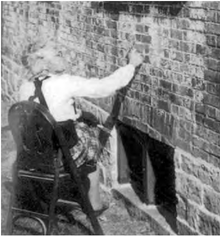
Betty scrapes old paint on the exterior brick by hand.
