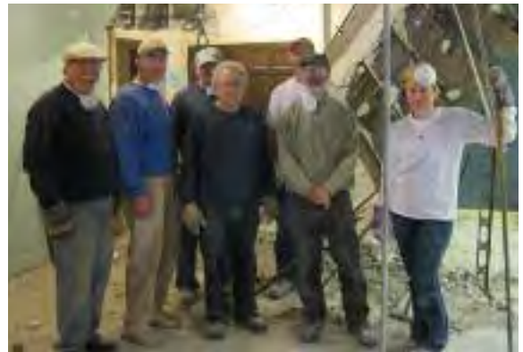
Volunteer crew who removed a wall in the theater lobby of the Riverside Arts Center.
