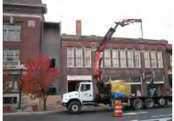
Boom truck delivering roofing materials last Friday.
